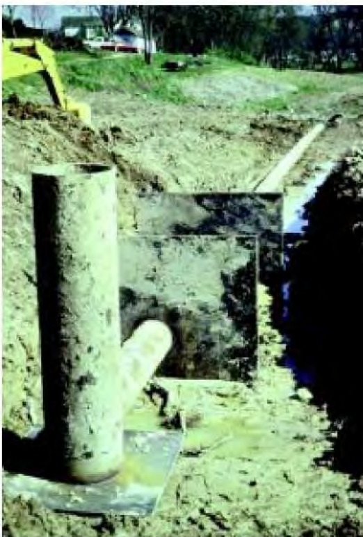
Figure 22 Drop-inlet pipe spillway with antiseep collar
